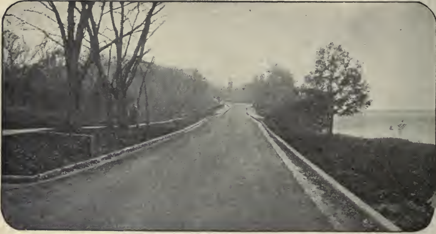
State Trunk Line No. 13 in Kilbourn, Wisconsin. Maintained with annual treatments of "Tarvia-B" since 1916
